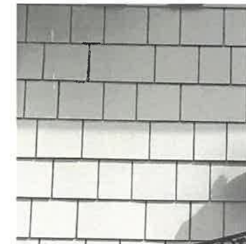
EXISTING SHAKE SIDING
