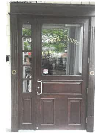
EXISTING FRONT DOOR
