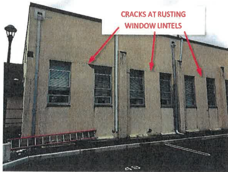
Photo 6 - Parish Hall Wall at Left Side, Facing North-West
