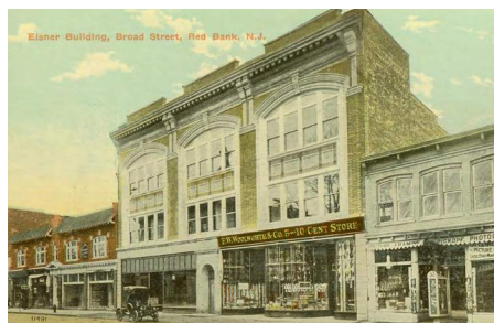
Eisner/Woolworth Building | 52 Broad St
