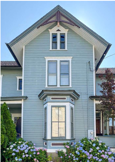
Tall, narrow double-hung windows with segmental arched hoods and a projecting bay.
