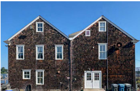
Side-gable roof with wood shingles, representative of early vernacular construction.
