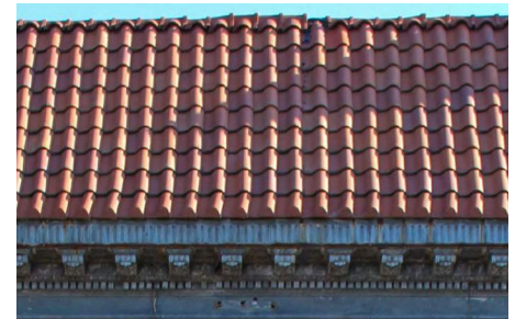
Clay barrel tile roof with ornate cornice showing rare influence of Mediterranean Revival style.
