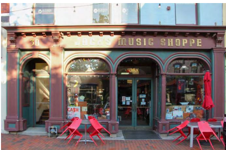
Rehabilitation preserving original arched openings, cornice, and storefront framing.
