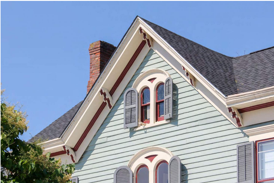
Steeply pitched cross-gable roof with open eaves and paired brackets, characteristic of the Gothic Revival style, with a corbeled-cap brick chimney.
