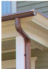
Copper U-style gutter.
