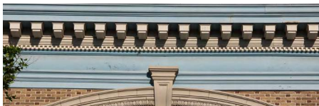
Classical wood cornice with dentils and deep overhang.
