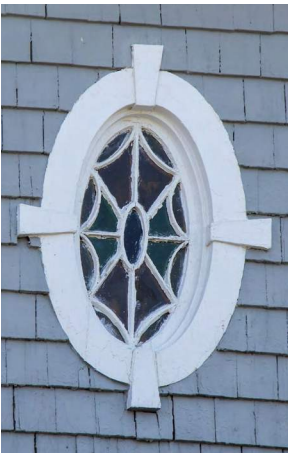
Leaded oval window with cross-shaped muntin detail, typical of Queen Anne.
