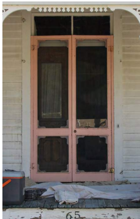
Historic wood-framed screen doors.
