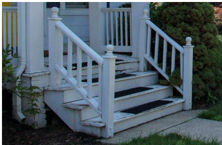
Simple wooden stairs with square newel posts and traditional balusters.
