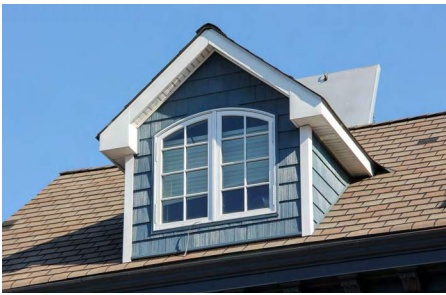
Contemporary front-gable dormer with arched multi-pane window and shingle siding.
