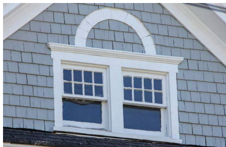
Paired double-hung windows with multi-pane upper sash and a decorative arched pediment.
