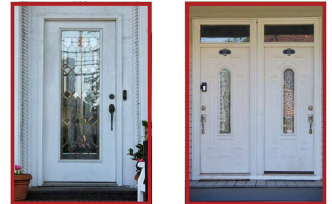
X Inappropriate Contemporary replacement front doors
