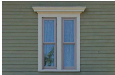
Pair of double-hung windows with simple crown molding
