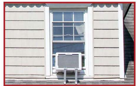
✗ Inappropriate Vinyl windows and air conditioner on primary façade.
