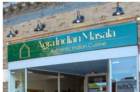
Gooseneck sign lighting fixtures mounted above a projecting signboard
