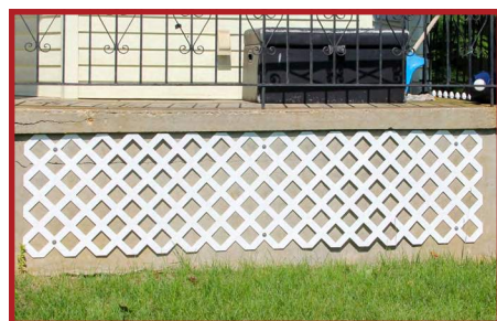
✗ Inappropriate Oversized plastic lattice over a concrete foundation.
