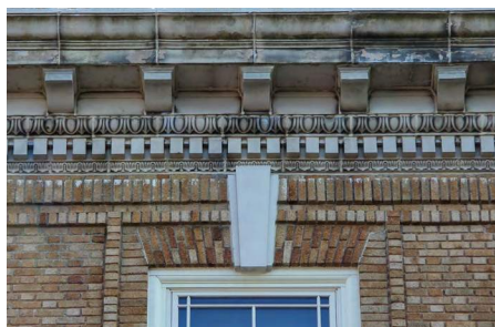
Brick with cast stone cornice and dentil detail, combining masonry and ornamental trim.
