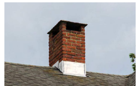
Chimney with bright metal flashing and simple cap
