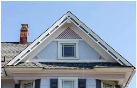
Staggered butt and diamond-pattern shingles.
