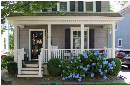
Porch with square columns, and simple balustrade
