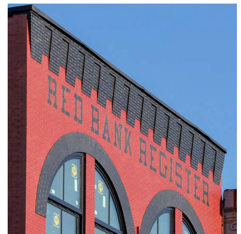
Corbeled brick cornice with stepped battlements and painted sign panel.
