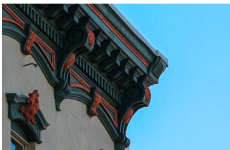
Italianate-style metal cornice with heavy brackets and applied roundels.
