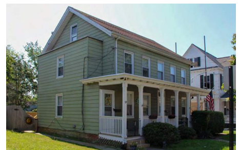
Side addition and porch extension
