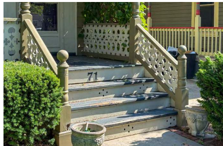
Sawn baluster stair with decorative caps and painted treads.
