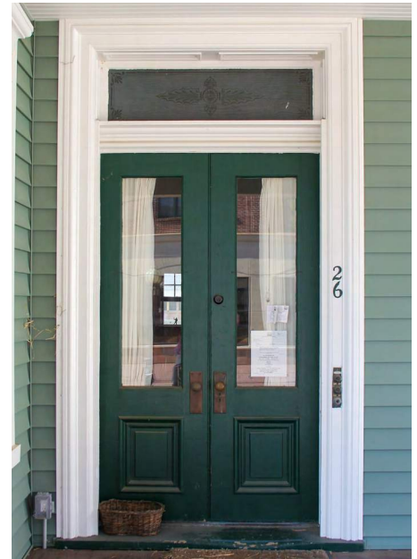
Traditional double doors with raised panels and glazed upper sections with transom.
