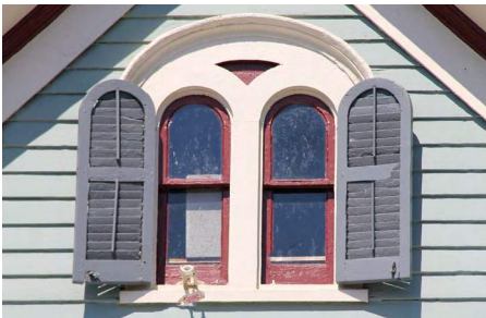
Paired arched windows with decorative trim and operable louvered shutters.
