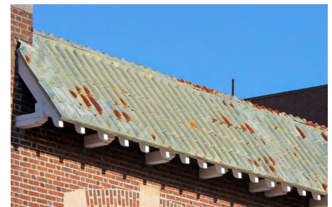
Front-gable metal roof with deep eaves and classical cornice returns.
