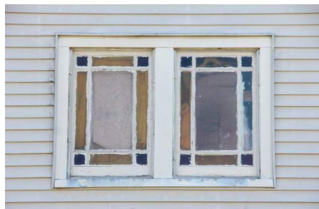
Art glass casement windows with geometric stained glass borders.
