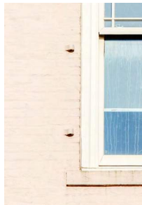
Intact pintle hinges can be used to indicate windows historically had shutters installed.
