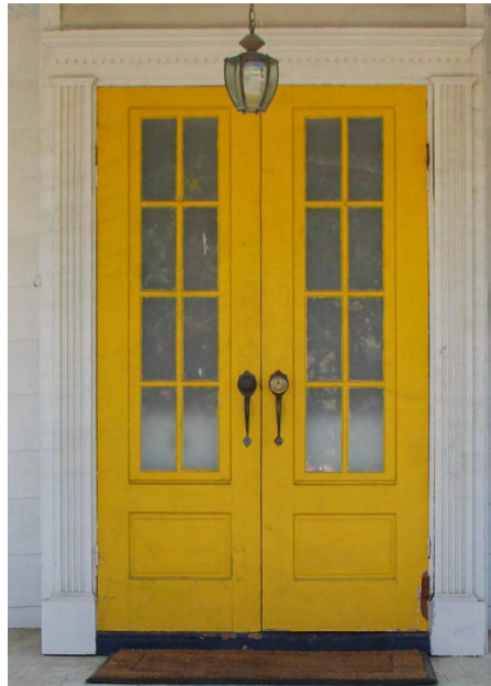
Full-light glazed double doors with divided panes and transom, accentuated by pilasters.
