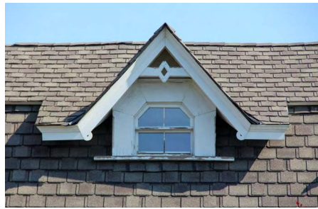
Decorative gable dormer with diamond-shaped gable vent and polygonal window frame.
