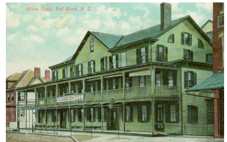
Globe Hotel, 1910 (partially demolished)
