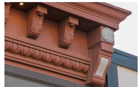
Ornamental wood cornice with rounded modillions over egg and dart molding.
