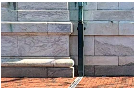
Stone cladding above water table foundation molding.
