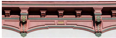
Decorative wood cornice with paired brackets and applied ornament.
