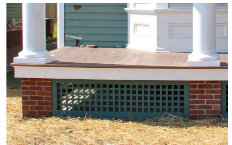
Eatlake-style piered balustrade (top) Brick piers with framed lattice between (bottom)
