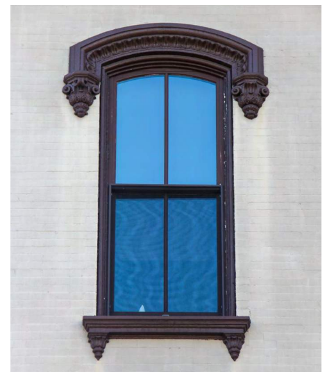
Round-arched window with elaborate molded hood, scroll brackets, and decorative keystone.
