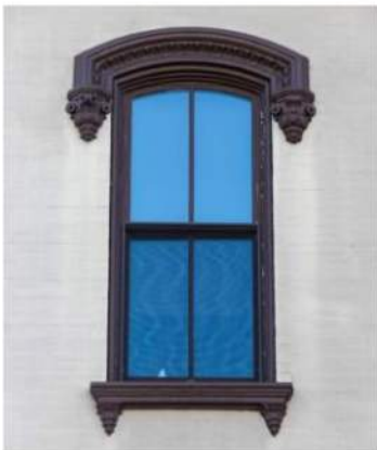
Round-arched window with elaborate molded hood, scroll brackets, and decorative keystone.
