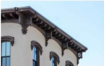
Bold Italianate cornice with paired brackets, deep eaves, and decorative cross-bracing at corners.
