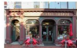
Rehabilitation preserving original arched openings, cornice, and storefront framing.
