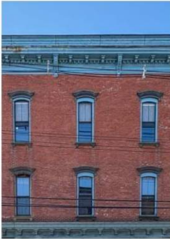
Segmental arched masonry window openings, common in Italianate buildings.
