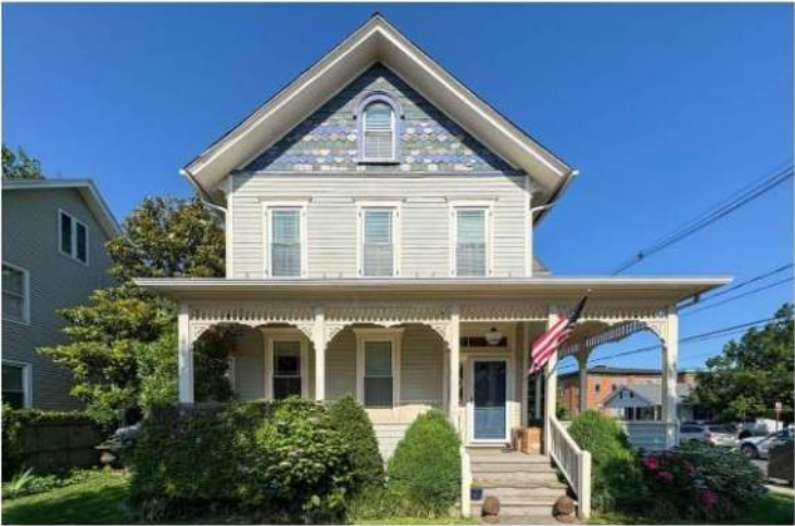
Wood siding on the main wall surface with decorative fish-scale shingles in the front-facing gable, combining texture and color variation typical of late 19th-century Victorian-era design.
