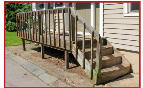
✗ Inappropriate Unpainted pressure-treated lumber stair and railing.
