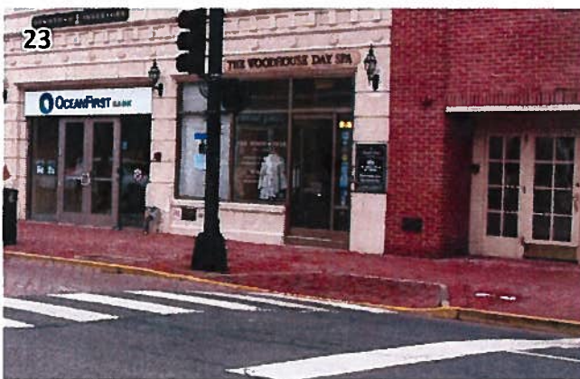
23 The northern half of Broad St is finished with brick paver sidewalks that are generally in good condition. Brick paver curb ramps should be retrofitted with detectable warning surface. (RedBank_180201_093350.JPG, RedBank_180201_093439.JPG)
