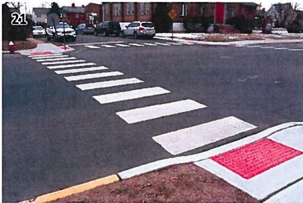
21 The intersection of Bridge Ave and Herbert St is an excellent example of ADA compliant curb ramps and high visibility crosswalks that could be replicated throughout the borough. (RedBank_180201_084125.JPG)
