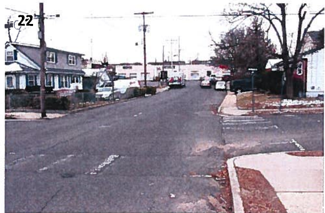
22 The intersection of Drummond Ave and S Bridge Ave is an example of an intersection due for curb ramp replacement and crosswalk re-stripping. (RedBank_180201_084825.JPG)
