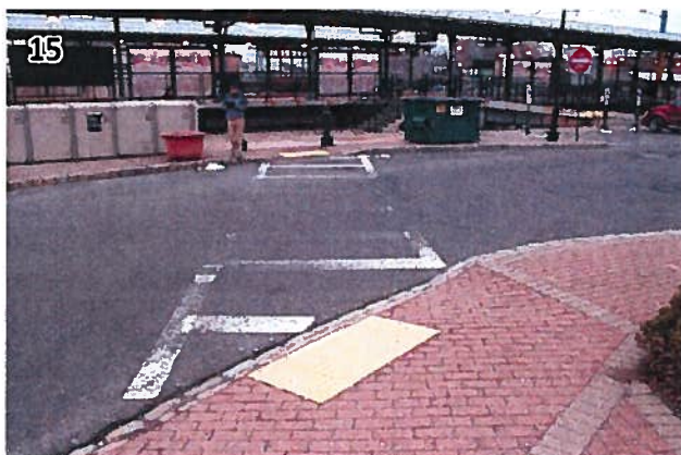
Cars were observed moving quickly through the station area. It may be advisable to post a parking lot speed limit (such as 9 MPH) and increase the visual presence of pedestrian crossings. (RedBank_180201_073921.JPG)
