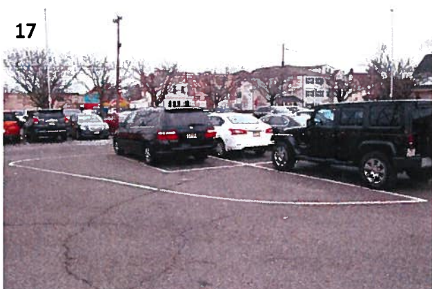
Lot 03 includes striped parking lot islands. These can be retrofitted as infiltration gardens through pavement removal, curbing, soil amendment, and planting. (RedBank_180201_074922.JPG)
