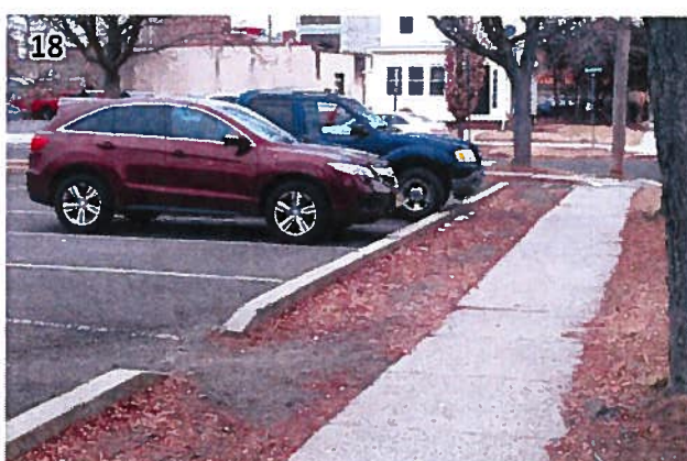
The eastern edge of Lot 03 could be retrofitted with a bioswale between the parking lot and sidewalk to aid in stormwater infiltration. (RedBank_180201_075201.JPG)
