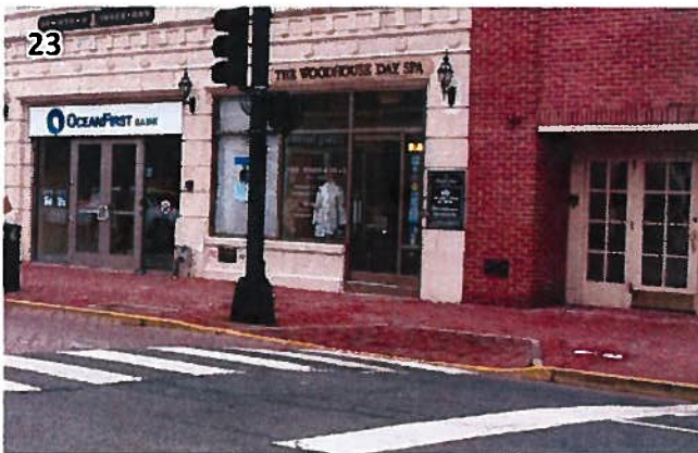
23 The northern half of Broad St is finished with brick paver sidewalks that are generally in good condition. Brick paver curb ramps should be retrofitted with detectable warning surface. (RedBank_180201_093350.JPG, RedBank_180201_093439.JPG)
