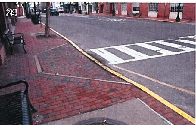
23 The northern half of Broad St is finished with brick paver sidewalks that are generally in good condition. Brick paver curb ramps should be retrofitted with detectable warning surface. (RedBank_180201_093350.JPG, RedBank_180201_093439.JPG)
