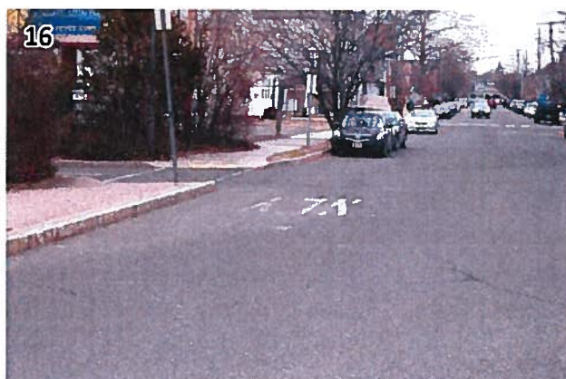
Markings and striping throughout the parking lots are due for replacement. (RedBank_180201_074611.JPG)
