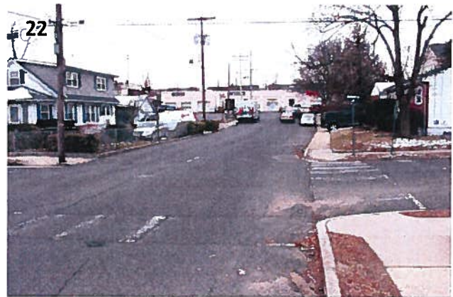
22 The intersection of Drummond Ave and S Bridge Ave is an example of an intersection due for curb ramp replacement and crosswalk re-striping. (RedBank_180201_084825.JPG)
